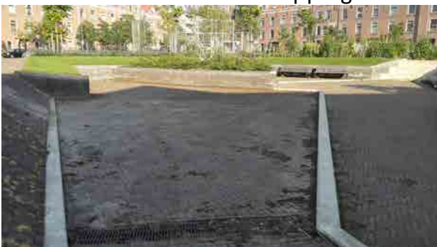
Figure: Bellamyplein in dry situation, there are a lot of residue on the pavement. Source: author
