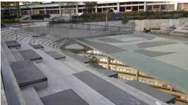
Figure: Benthemplein after rain, a playground for dry situation. Source: author
