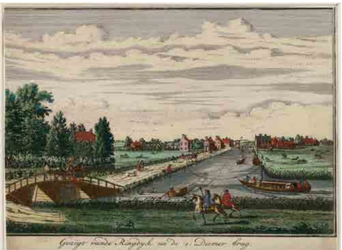
Figure 20 Outer-ring canal 1725, People has leisure activities along the ring canal
