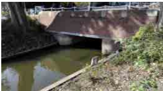
Figure 42 Bridge on internal channel with Amsterdam School style
